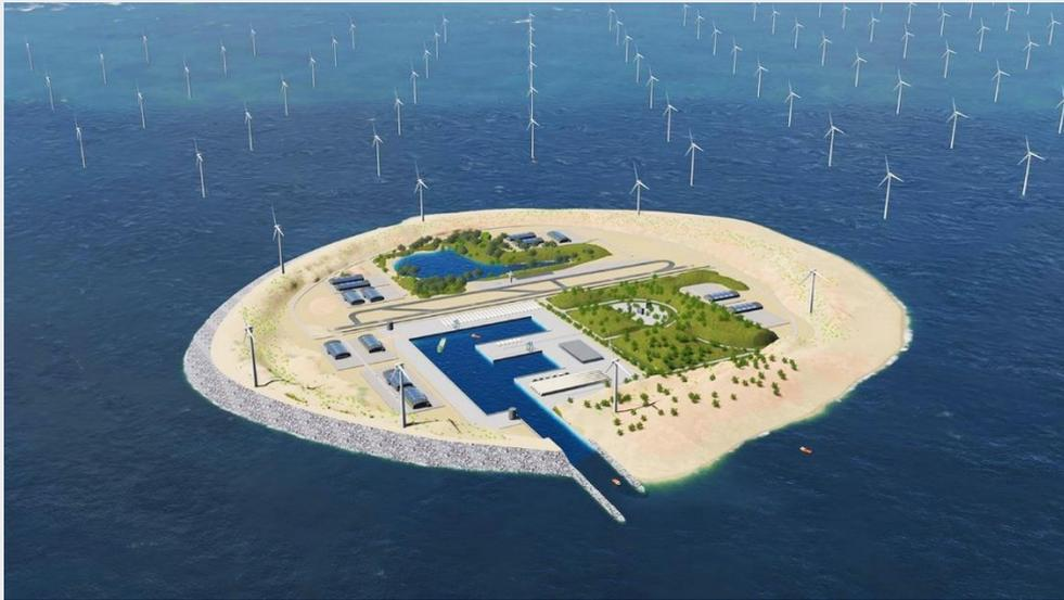
Figure 2 Impression of an artificial island in the North Sea, fit to facilitate installation and O&M activities.
